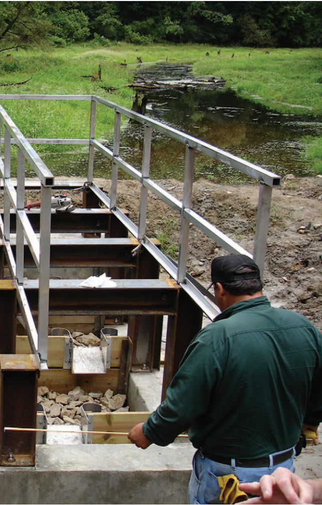
LEFT: This first-of-its-kind water control device allows for upstream migration of fish into Big Marsh Lake, a 200-acre shallow wetland that is part of Michigan Audubon's Bernard W. Baker Sanctuary in Calhoun County. © 2009 Jonathan E. Lutz. RIGHT: Cranes © Cory Gildersleeve, 2006.
